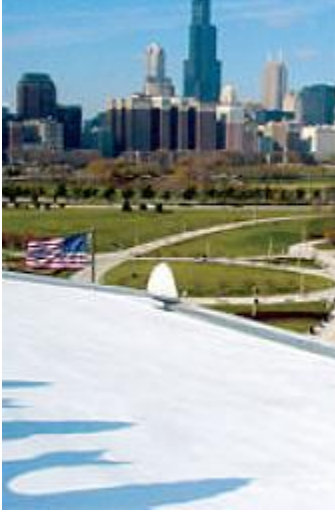
Chicago's Shedd Aquarium installed a white roof made of soy oil polymer in 2004. (Photo credit unknown)
