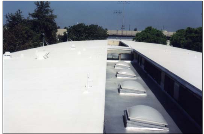
Advanced coatings Acu-Flex material was used on this school roof. The coating will block 100% of ultraviolet light and the roof will stay 85% reflective, even after 3 years.
